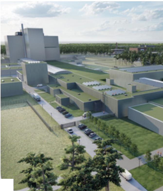
The MYRRHA reactor being built in Belgium will test accelerator-driven nuclear fission.
